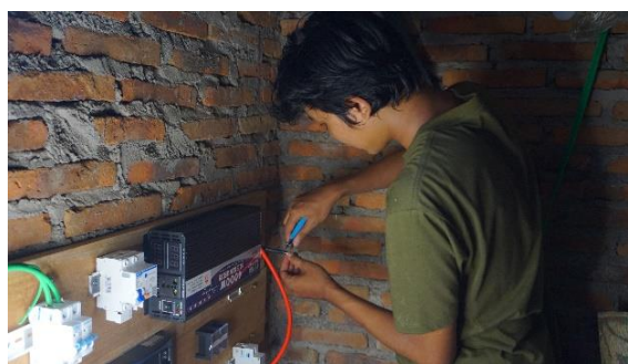
Gambar 10. Proses instalasi Controller
