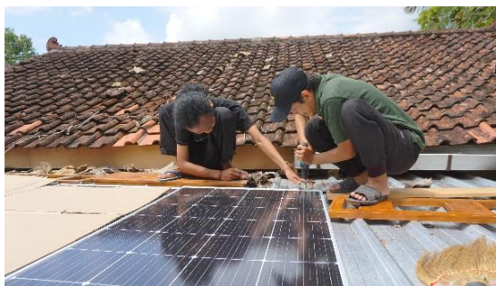
Gambar 8. Proses instalasi panel surya
